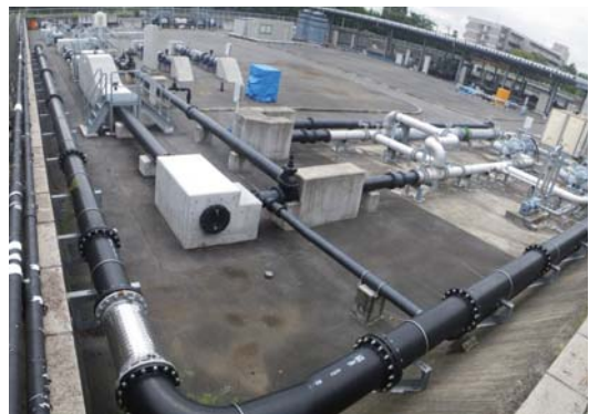
The development field with basic facilities for R&D such as loop pipes and pumps
