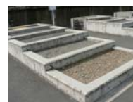
⑧ Cutaway model of different pavement types
