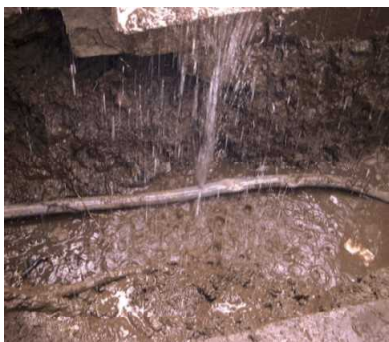
A leaking lead pipe
