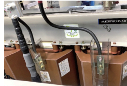
High-efficiency transformer (Yakumo Water Supply Station)
