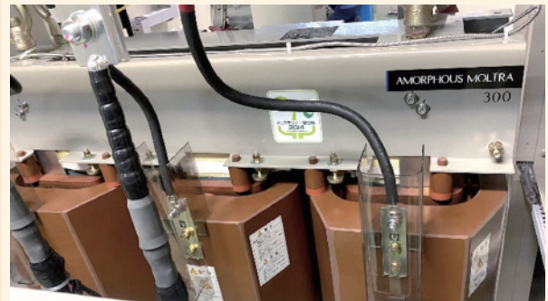
High-efficient transformer (Yakumo Water Supply Station)
