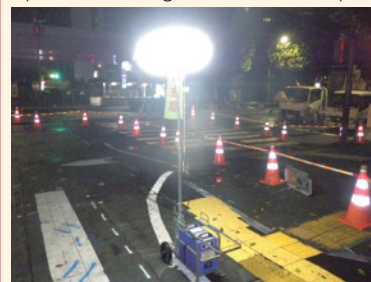
Noise control measures by battery-powered generator (Example of commendation)
