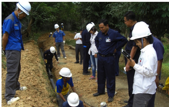
Figure 3.1 Replacements of Water Pipes as a Leakage Prevention Measure (In Yangon City, Myanmar; Japanese supervisor standing on the left)
