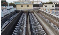
Fig. 8 Flocculators in the flocculation basin (Flame type)
