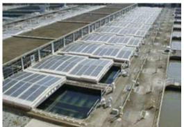
Figure 10: PV modules installed over filter basins
