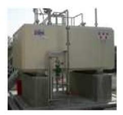
[Figure6] In-house power generation equipment and fuel tank
