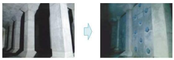
Figure 4: Earthquake resistance reinforcement work on the interior of a distribution reservoir
