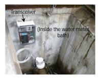
**Figure 10** Transceiver installation (Facility C)
