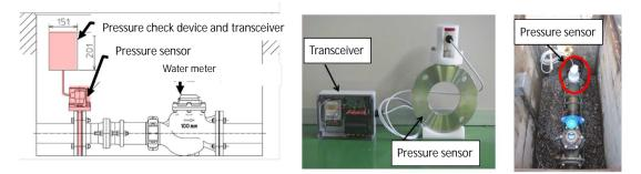
Figure 6 Structure of water supply pressure measurement points
