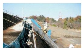
**Fig. 11**: Downstream slope preservation work (spraying thickening material)
