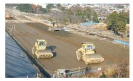
**Fig. 9**: Reinforcing embankment materials Levelling and compaction
