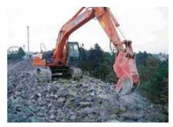
**Fig. 6:** Bomb-protection layer removal
