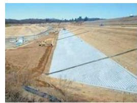
**Fig. 4**: Concrete blocks (Upstream side)
