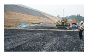
**Fig. 8**: Horizontal drain Levelling and compaction
