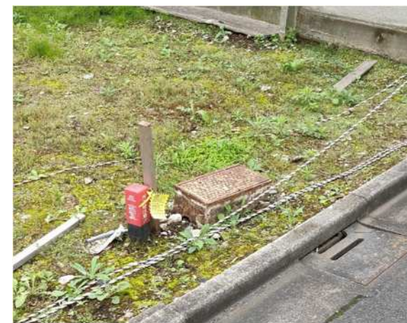
Fig.16 Service pipes not expected to be used
