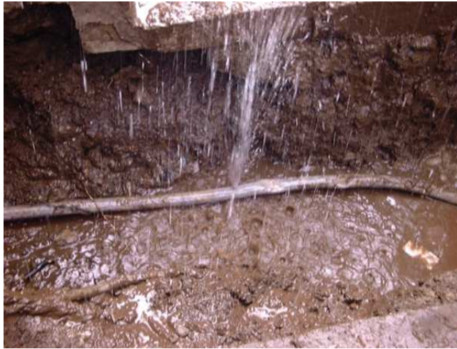
Fig.11 Leakage from lead pipes
