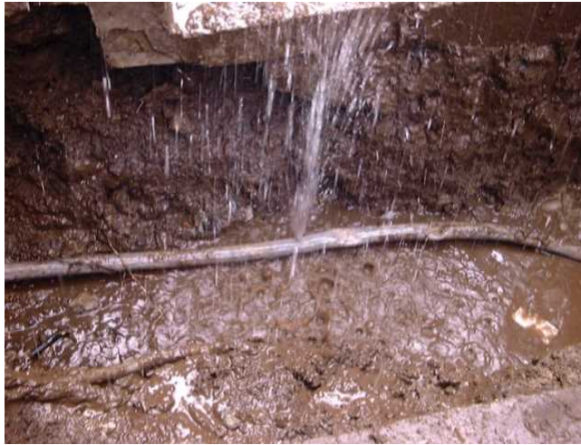
Fig.11 Leakage from lead pipes
