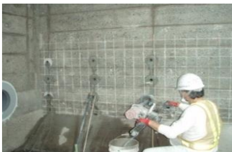
Figure 2. Sidewall boring
