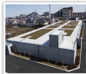
Rooftop greenery at Saiwaicho Water Purification Plant
