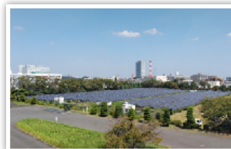
Solar Panel Facilities (Higashi-Murayama Purification Plant)
