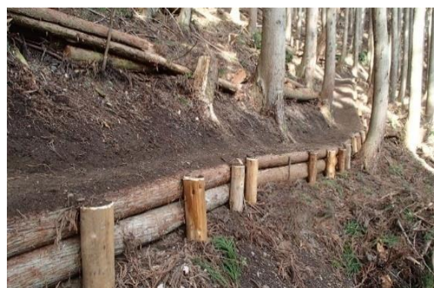
Maintaining a path for forest management (fence made from timber from thinning)
