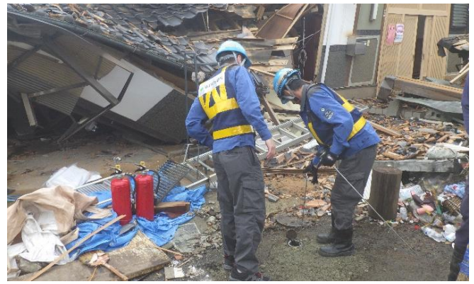
Survey on Water Leakage (The Kumamoto Earthquake) 漏水調査（熊本地震）
