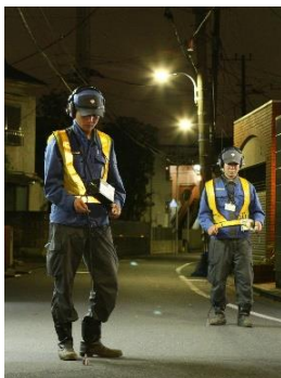
Leak Detection Work at Night 夜間の漏水調査作業
