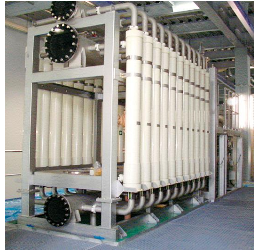
Membrane Filtration Facilities 膜ろ過設備
