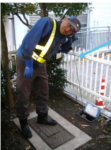
Leak Detection Using a Leak Sound Detection Bar
