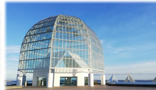
The Glass Dome of the present aquarium
