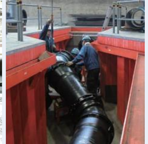
▲ Training to connect water pipes
