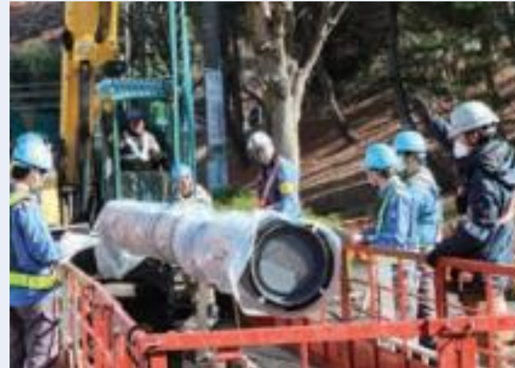
▲ Survey of detecting water leakage
