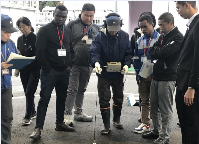
▲ Drill for water leakage investigation
