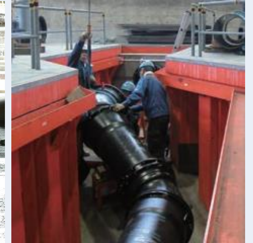
▲ Training to connect water pipes
