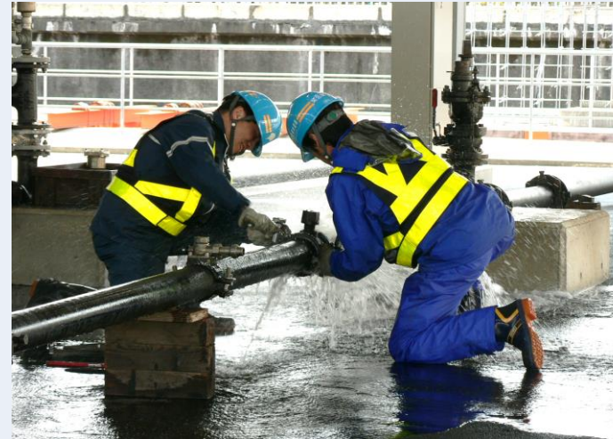
▲ Training to repair leaking water pipes
